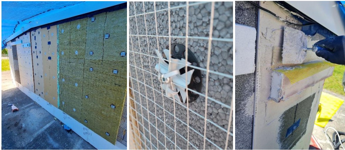
Figure 24: Insulated façade under scaffold sheeting before plastering (left); steel mesh for the thick plaster system and a mesh fastener on top of an insulation anchor (center); application of lime-cement (L/C) plaster and reinforcement profiles at the XPS corners on top of the EPS insulation (right).
