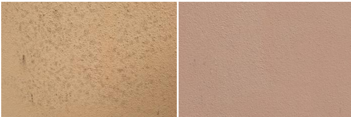
Figure 31: Biological growth on 25 March 2025 on the thick plaster (NHL system) on wood fibre board insulation all over the section on southern facade (left) and same area on 07 August 2025 (right). (Talvik et al., 2025)
