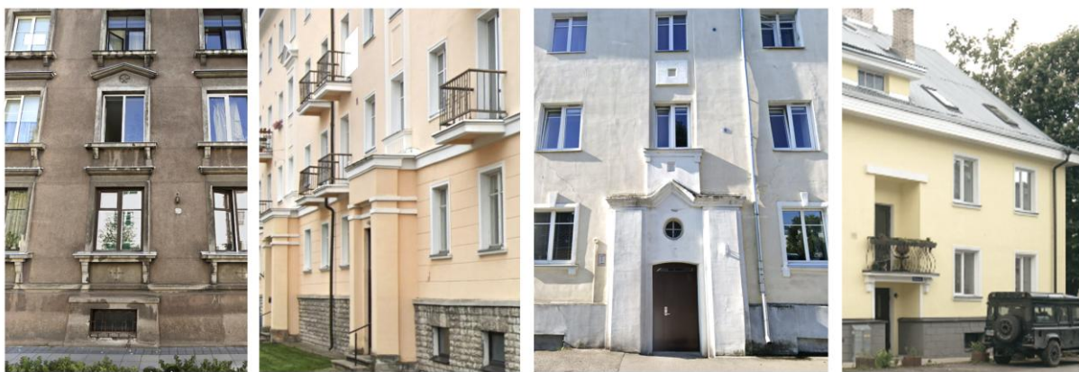
Figure 2: Examples of facade finish decor variations on the archetypical Stalinist brick apartment buildings (photos from left: Google StreetView, Paul Klõšeiko, Google StreetView, Paul Klõšeiko).
